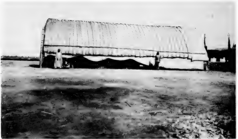
SHEIKH KHAZAL IBN FALIH'S GUEST HUT, CONSTRUCTED OF 150 REED MATS
